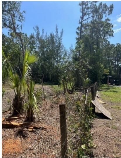
Figure 9. Canal 6 Bank After Vegetation Removal
